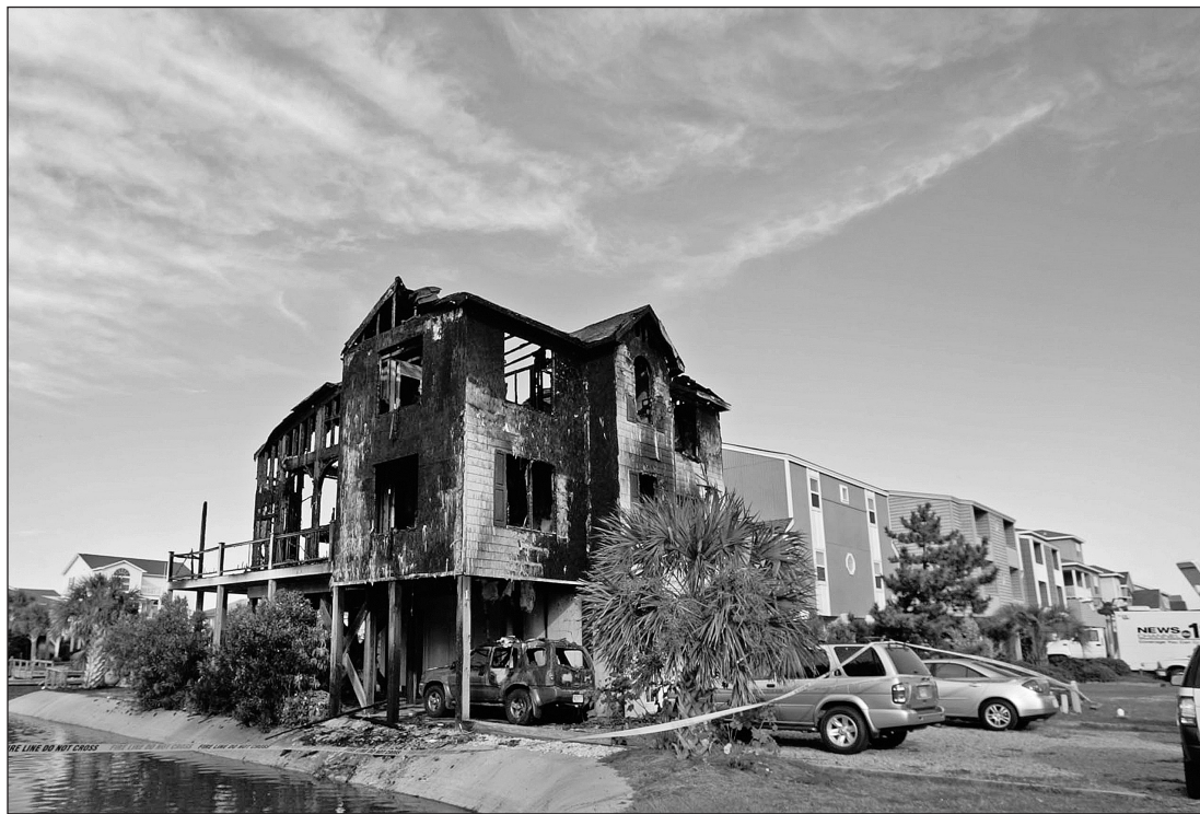
RANDALL HILL / Myrtle Beach Sun-News via MCT The burned remains of a home are seen Monday in Ocean Isle Beach, N.C. Seven were found dead after the fire, which officials say may have started on an outdoor deck.
