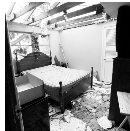
CHUCK BURTON / ASSOCIATED PRESS Pieces of the roof and ceiling lay on the floor of a bedroom in a damaged home in Vale, N.C., Wednesday, Oct. 27, 2010.
