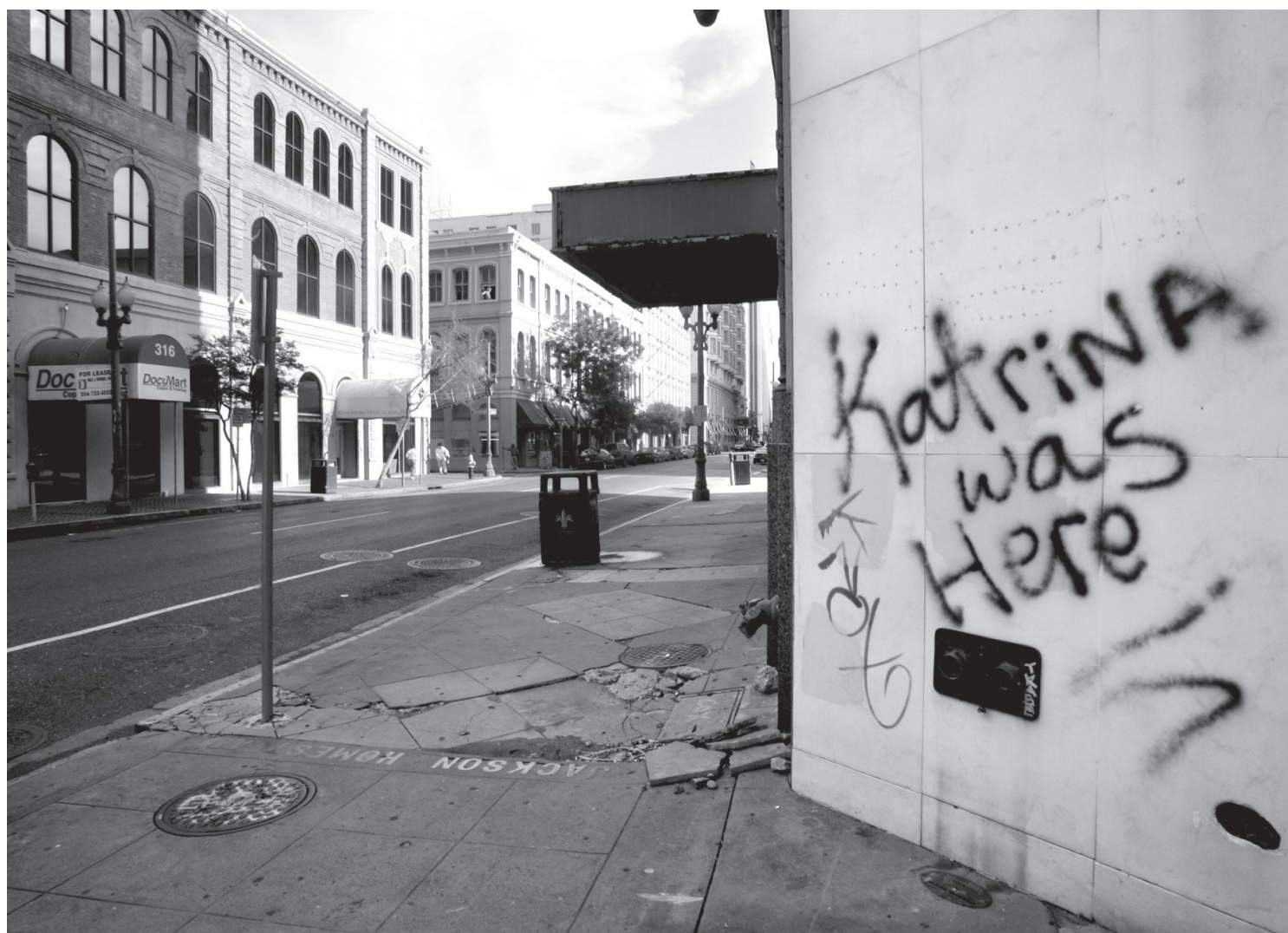
A message spray-painted on a building in downtown New Orleans in August 2005 was enough to explain what was responsible for the damage and the desolate streets. COURTESY OF MCT
