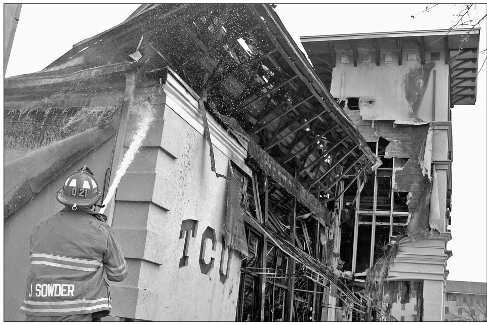
Capt. Jim Sowder of the Fort Worth Fire Department sprays water on the burned-out shell of the TCU Bookstore Wednesday to help prevent hot spots from re-igniting the blaze that consumed the structure that morning.
