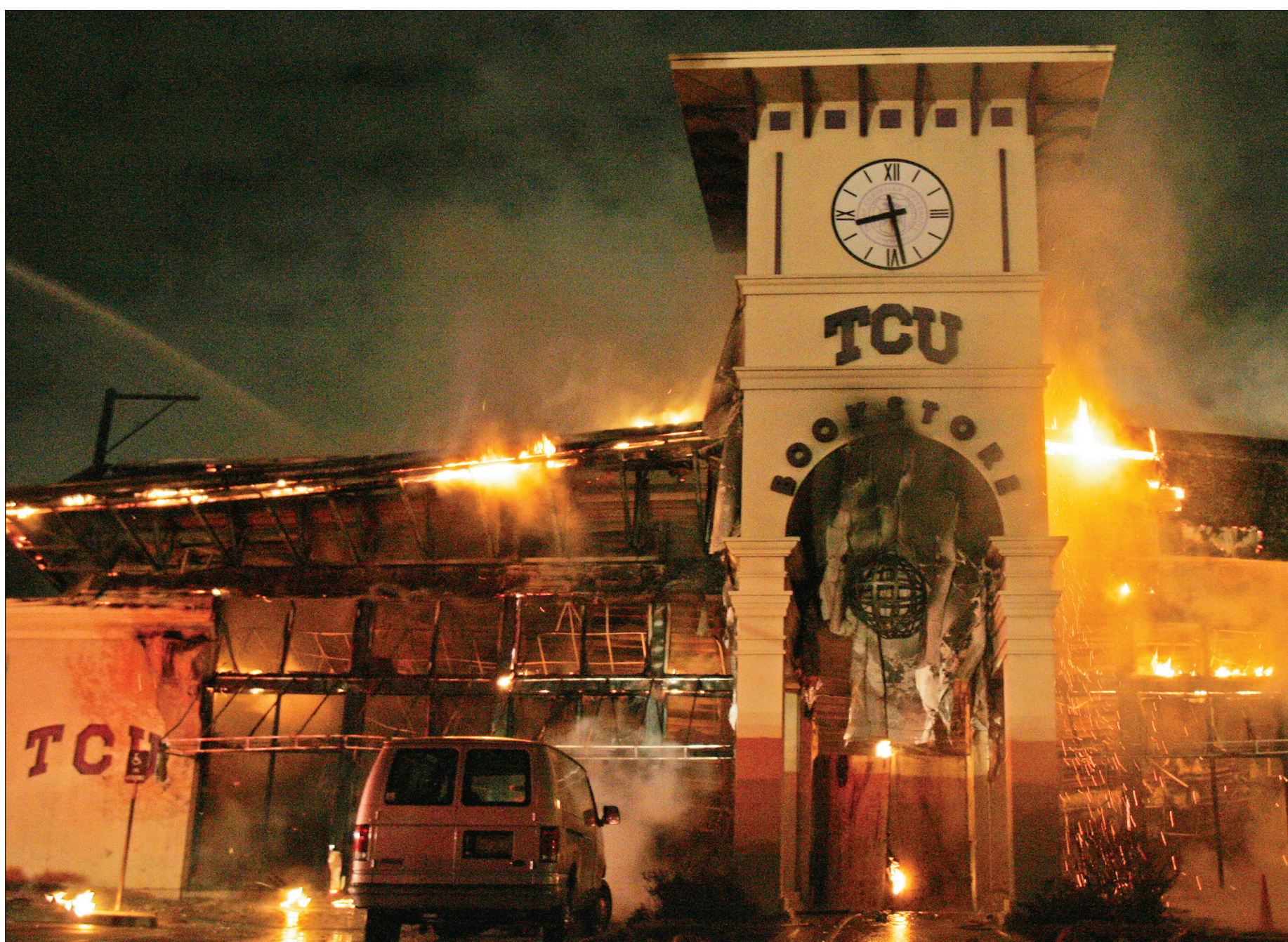
A fire broke loose Wednesday morning inside the TCU Bookstore at the corner of University Drive and Berry Street. The structure was in the process of renovation, and the fire caused an estimated $1 million in damage.
