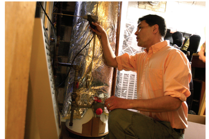
NANCE STONE / Chicago Tribune via MCT Wayne Yinger performs an energy audit at a home in Silver Spring, Md., on March 19.
