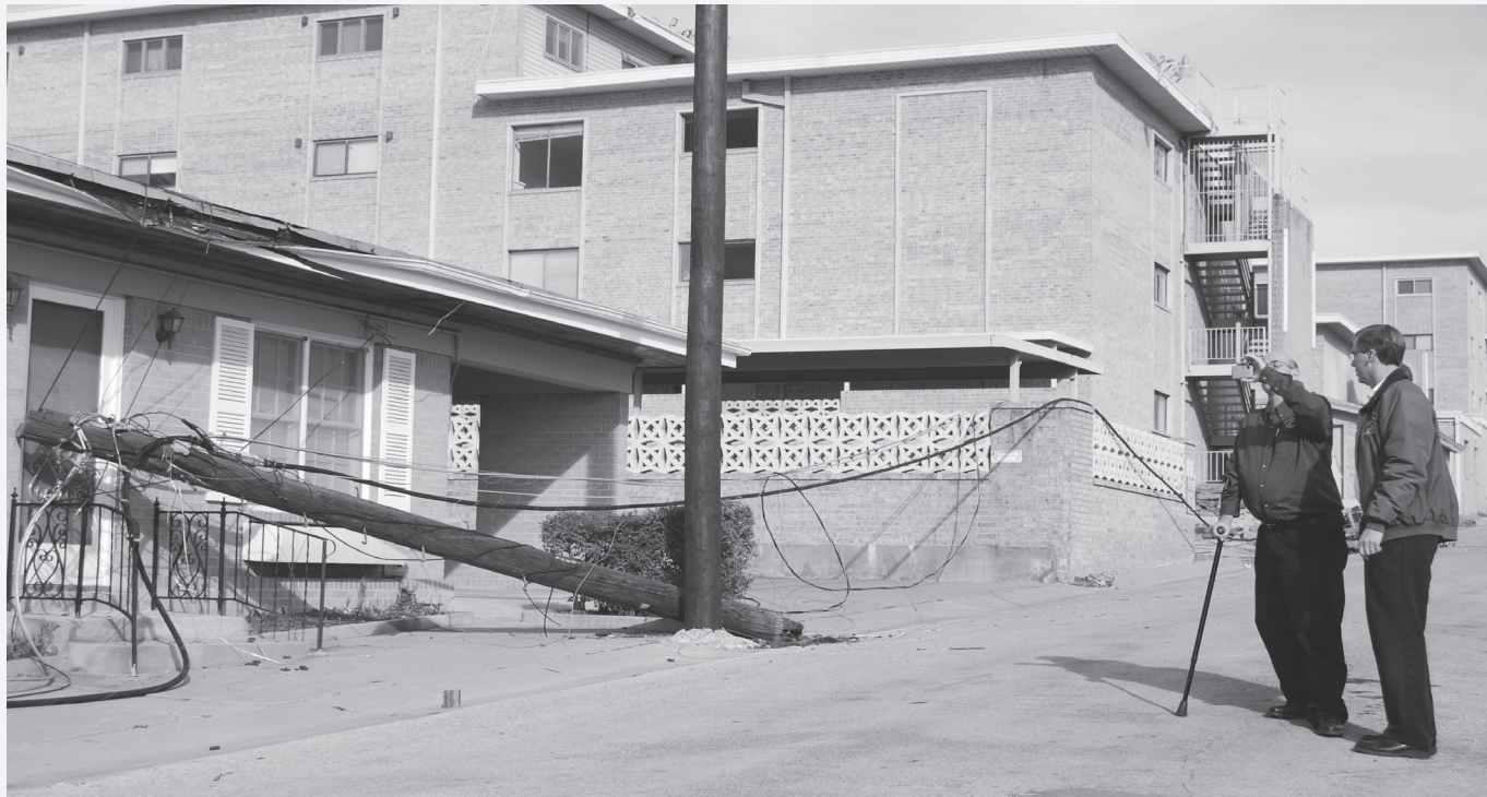
Randy Cobb, safety director at TCU Risk Management, investigates the site where a telephone pole crashed into a house on Pond Drive in Worth Hills. A delivery truck's top corner caught wires, dragging down two telephone poles and a smaller pole Tuesday, temporarily closing the street, according to TCU Police.
