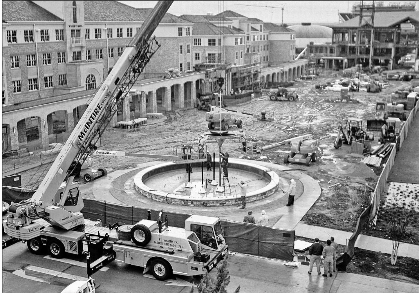
Workers assemble the refinished Frog Fountain on Dec. 12. Jef Larremore, the Web services coordinator for Student Affairs, watched the fountain go up last month and took this photo from the roof of the Brown-Lupton Student Center. To see more photos, visit the Skiff's newsroom blog at blogs.tcuailykskiff.com . If you have photos for the Skiff you can send them to yourtcu@dailykskiff.com .
